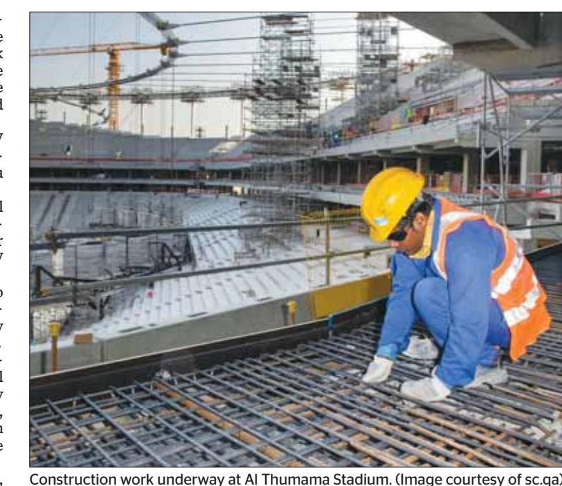
Construction work underway at Al Thumama Stadium. (Image courtesy of sc.qa)
